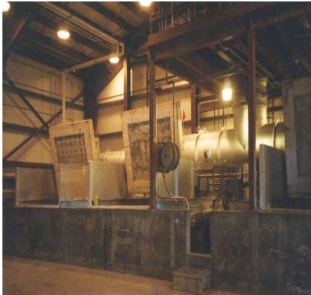
Waste Processing Modules
